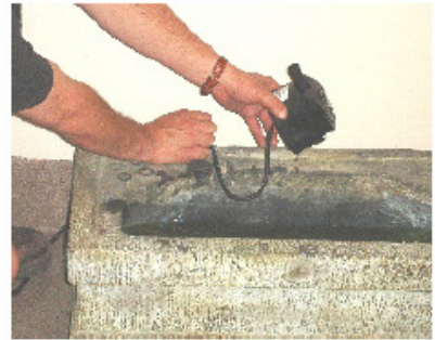
2) Place pump, with adapter, in basin. Cord loops out the back.
