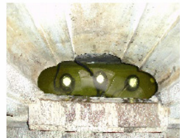
4) Install 3-Light Kit inside base and run cord out back.
