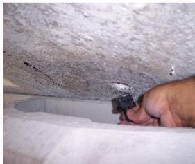
7. Thread the remaining adapter into the underside of the 4226B wall unit.
