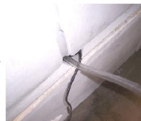
9. The clear tube and pump cord should exit the notch between the 6226 bowl and 4226B wall as shown. Shim as needed.
