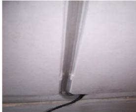
12. The clear tube should now rest inside the vertical groove behind the wall unit.
