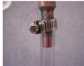
11. Push the top end of the clear tube onto the spray ring's entry pipe which is turned down behind the top of the wall.
