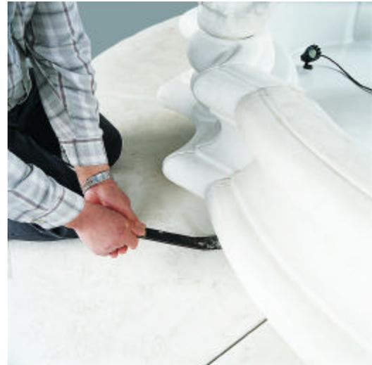
*Using a wide face pry bar to adjust wall sections*
